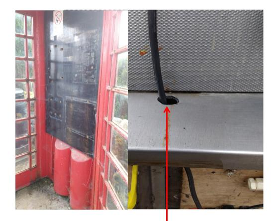
Beware sharp edges – use Rubber Grommet/Cable Gland on holes through metal
