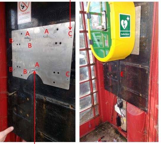
M10 bolts, configured here to fit a DefibSafe2
